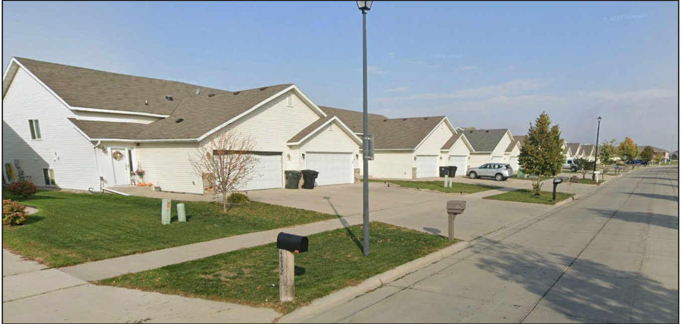
Above: Complete sidewalks and density support walkability in this twin home development, but design is still geared toward vehicle traffic, as evidenced by the row of wide driveways and front-loading garages. (Image Source: Google Earth)
