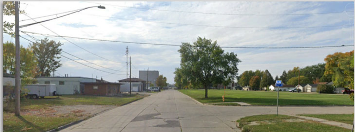
Dyke Avenue looking west toward UND. Aging properties and vacant space show this area's revitalization potential. (Image source: Google Earth)
