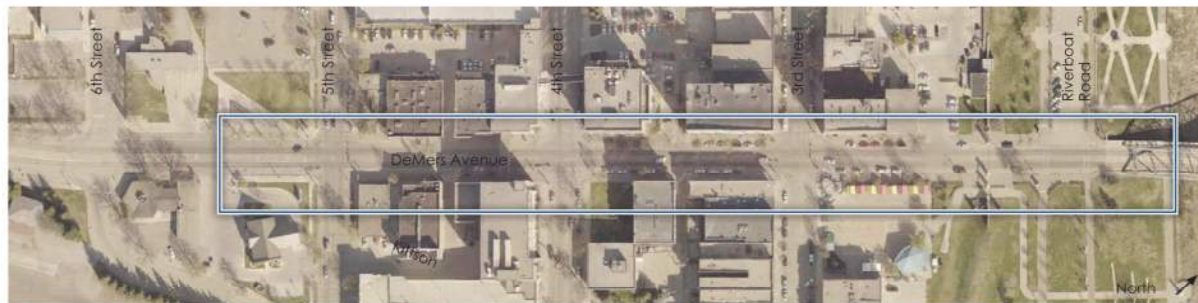
DeMers Avenue Overpass Bridge
