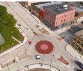
6th St N Mini-Roundabouts (GF)
