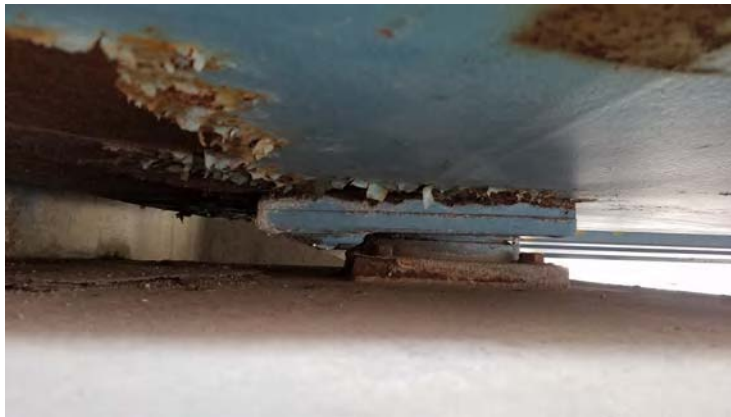
Figure 8 – Bearing at North Abutment under Girder No. 1 (West Fascia Girder)
