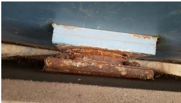
Figure 6 - Bearing at North Abutment under Girder No. 3
