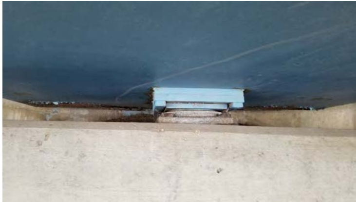
Figure 9 – Bearing at North Abutment under Girder No. 2. Note bars on sides of sole plate that provide lateral restraint.
