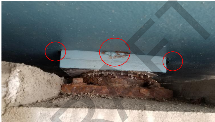
Figure 7 - Bearing at North Abutment. Girder No. 4 Note notch cut into top of pedestal because pedestal was cast too tall. Also note failed paint coating in vicinity of welds between sole plate and girder flange.
