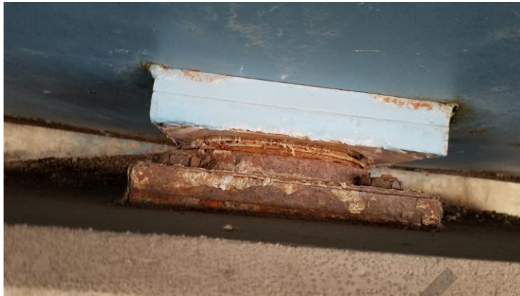
Figure 6 - Bearing at North Abutment under Girder No. 3
